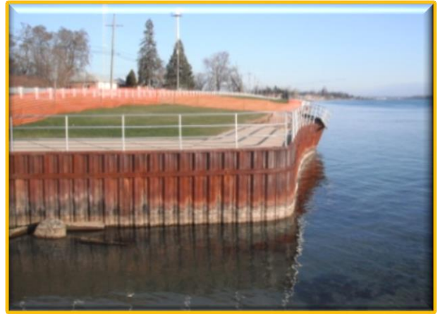
Failing seawall and sidewalk poses a safety risk
